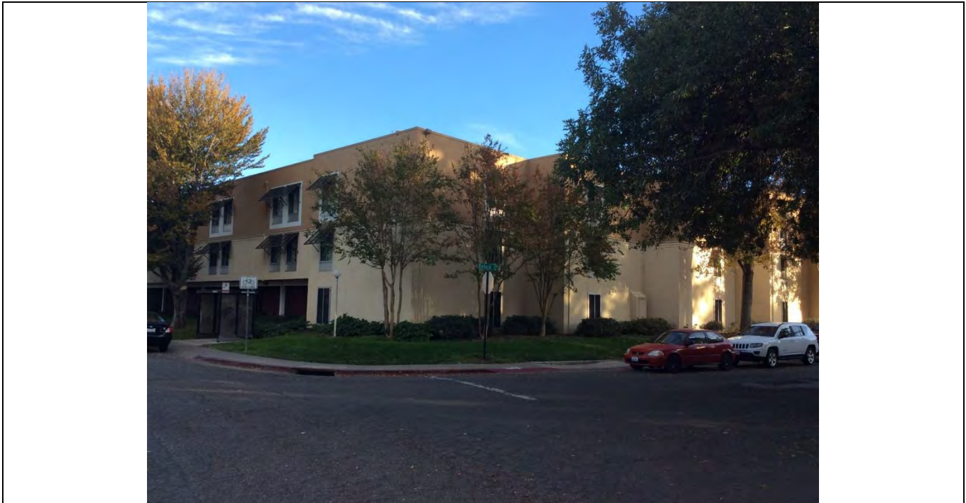
Figure 15. North and West Elevations, Displaying Sawtooth “Stepping” on West Elevation (Right), View to Southeast; November 14, 2017 (IMG_0801)
