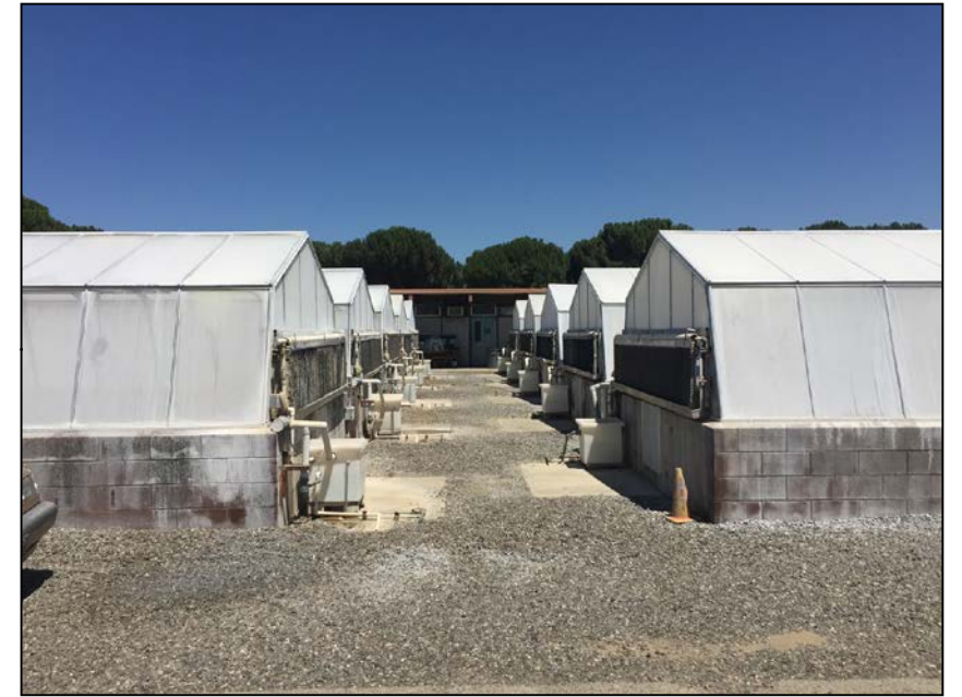
Orchard Park greenhouses site
