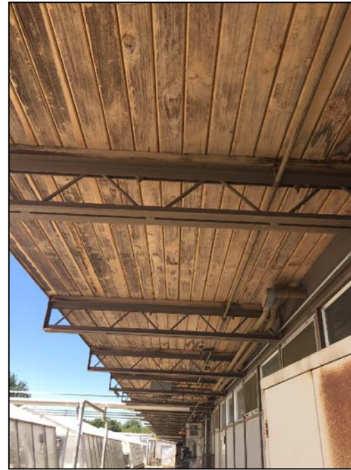
Typical roofing on Orchard Park greenhouses building
