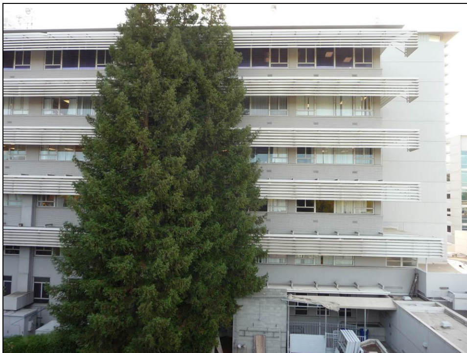
Photograph 7: Front (west) façade, south end. Note cast concrete spandrels, window arrangement, and metal louvers. Camera facing east, October 22, 2014.
