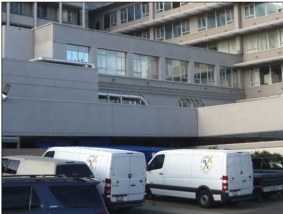
Photograph 12: Detail of wing on the east side of the north end of the North-South Wing that was original to 1929 administration building. Third floor added when North-South Wing was constructed. Camera facing southwest, October 22, 2014.
