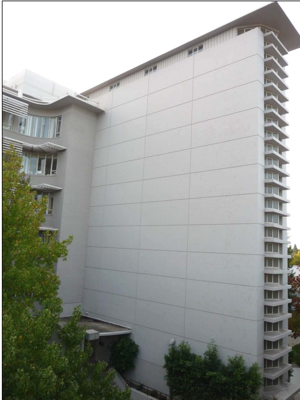
Photograph 4: Projection on front (west) façade of North-South Wing that houses an interior ramp. Note texture and pattern of exterior walls. Camera facing southeast, October 22, 2014.
