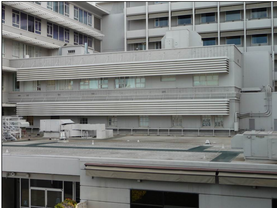
Photograph 11: Detail of wing on the east side of the south end of the North-South Wing that was original to 1929 administration building. Third floor added when North-South Wing was constructed. Camera facing north, October 22, 2014.
