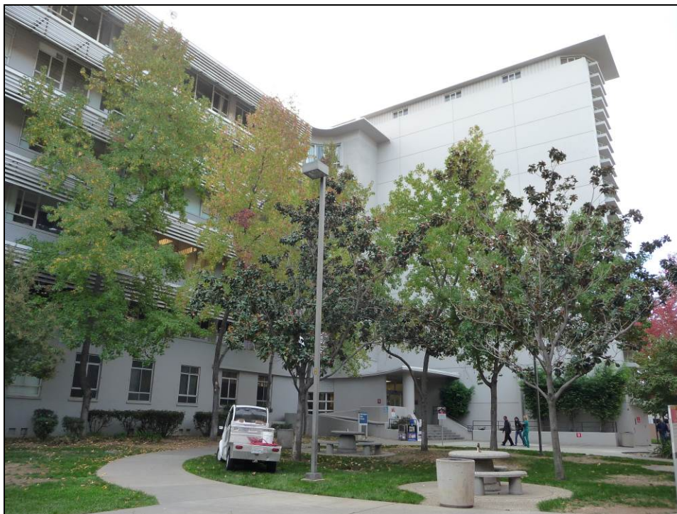
Photograph 8: Front façade (west) North-South Wing. Note windows on ground level. Camera facing southeast, October 22, 2014.
