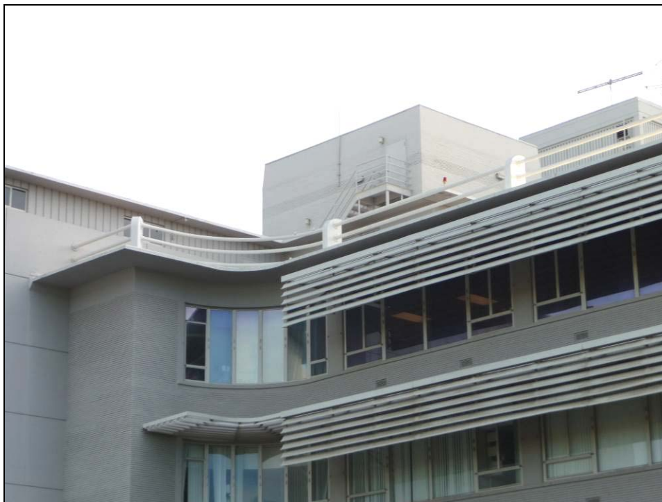
Photograph 5: Front façade, North-South Wing,. Note penthouse level at left connecting to components atop main roof. Camera facing northeast, October 22, 2014.
