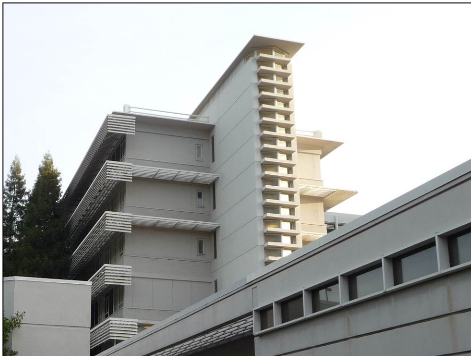
Photograph 2: South end of the North-South Wing. Note narrow projection that houses an interior stairwell and repetitive window detail at the end. Camera facing north, October 22, 2014.
