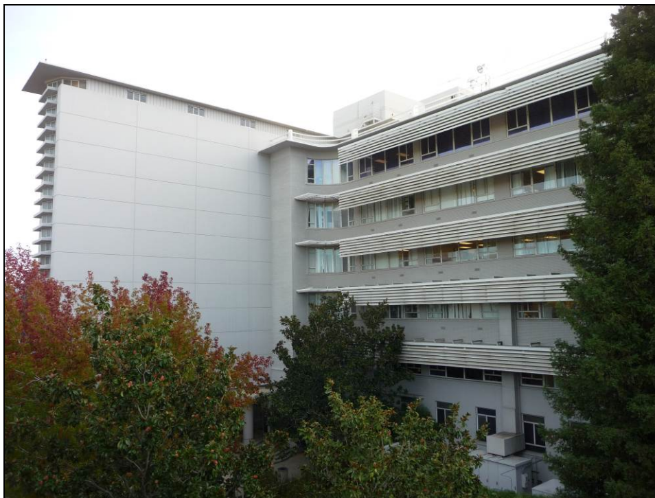
Photograph 6: Front (west) façade, North-South Wing. Note rounded junction with westward projection. Camera facing northeast, October 22, 2014.
