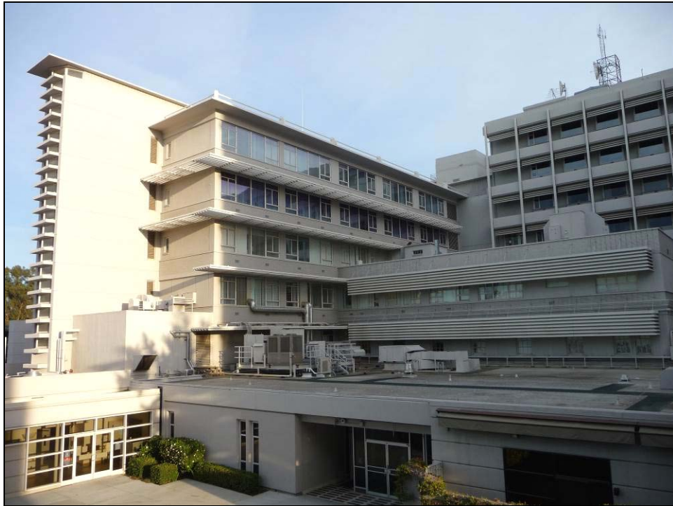
Photograph 10: South end of rear (east) façade North-South Wing. Note three-story perpendicular wing. Camera facing northwest, October 22, 2014.
