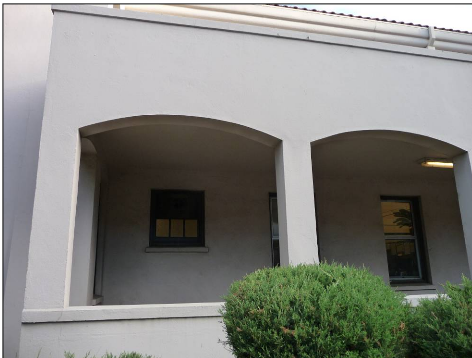
Photograph 5: Window at left front (south) façade is only original window remaining in Housestaff Facility. Camera facing north, October 22, 2014.
