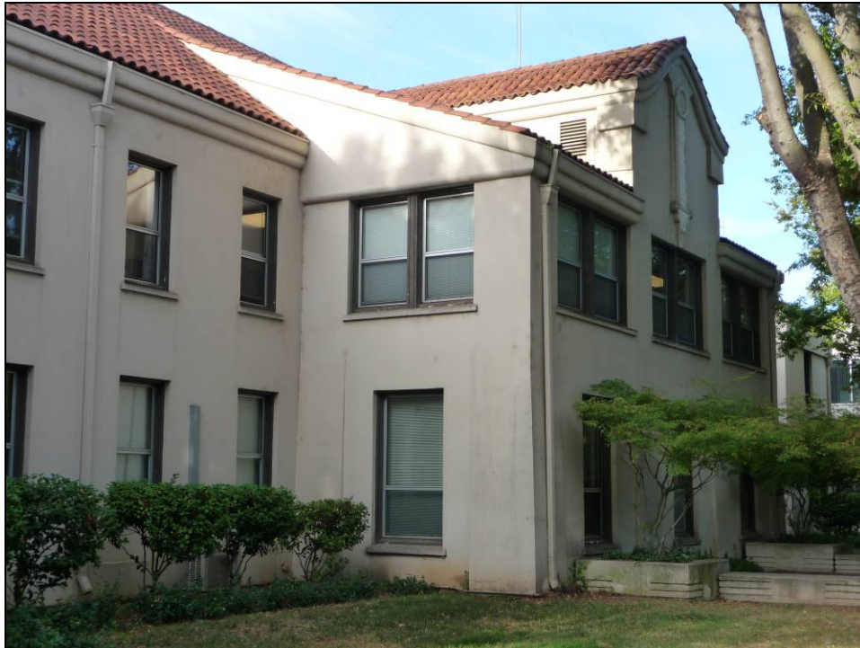
Photograph 8: Central projection of rear (north) side of Housestaff Facility. Camera facing southwest, October 22, 2014.
