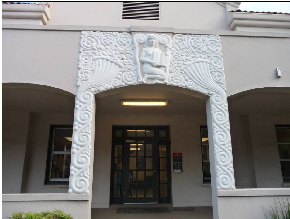
Photograph 4: Detail of cast-concrete panel and main entry on front (south) façade. Camera facing north, October 22, 2014.
