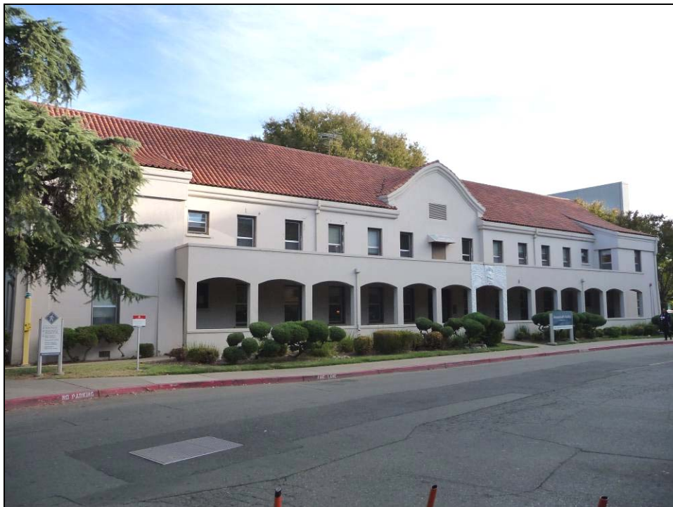
Photograph 3: Front (south) façade of the Housestaff Facility. Camera facing northwest, October 22, 2014.
