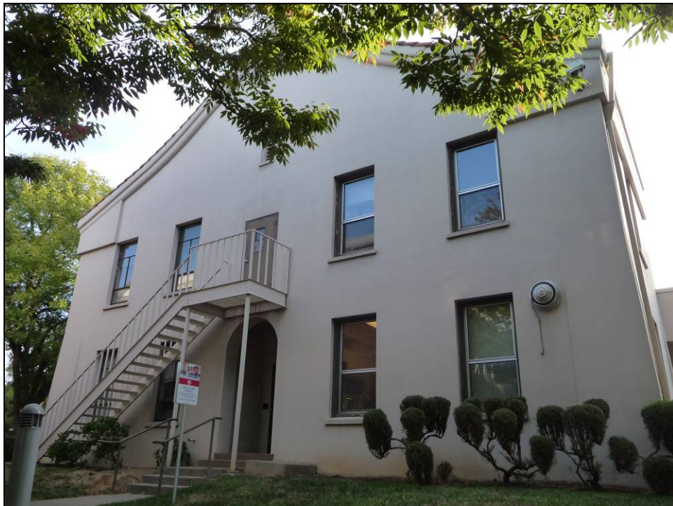
Photograph 7: South end Housestaff Facility. Note two generations of replacement windows, one on each side of staircase. Camera facing southwest, October 22, 2014.
