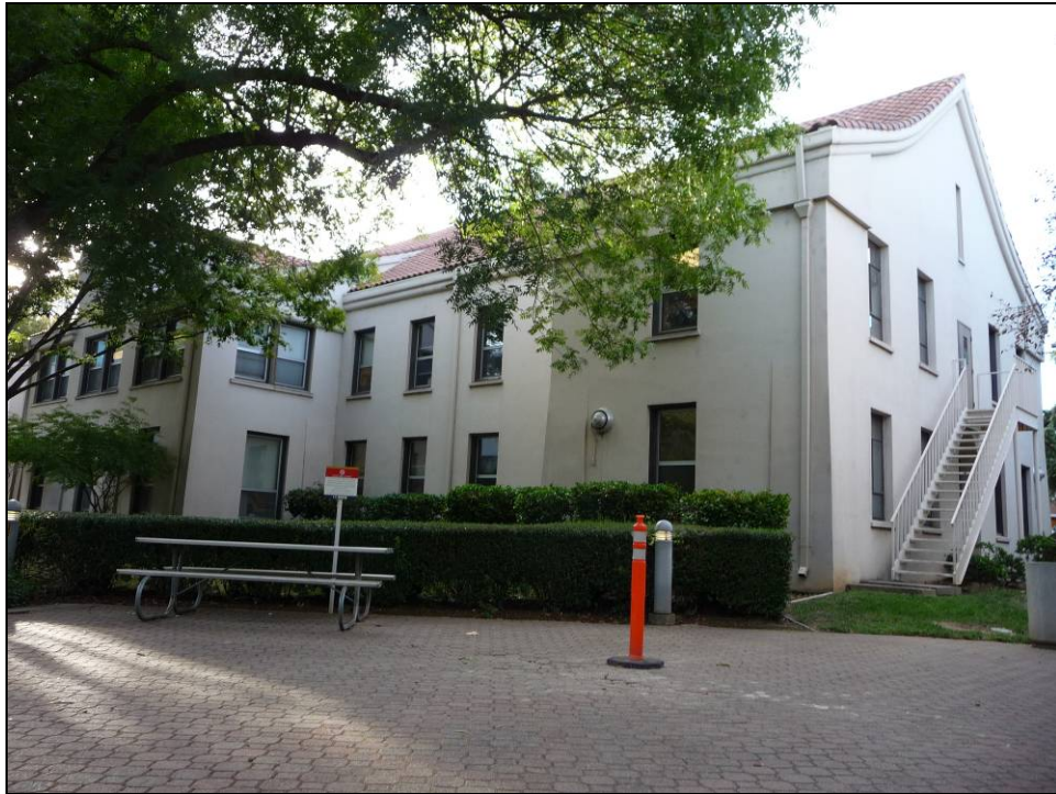
Photograph 6: North end of Housestaff Facility at right. Camera facing southeast, October 22, 2014.
