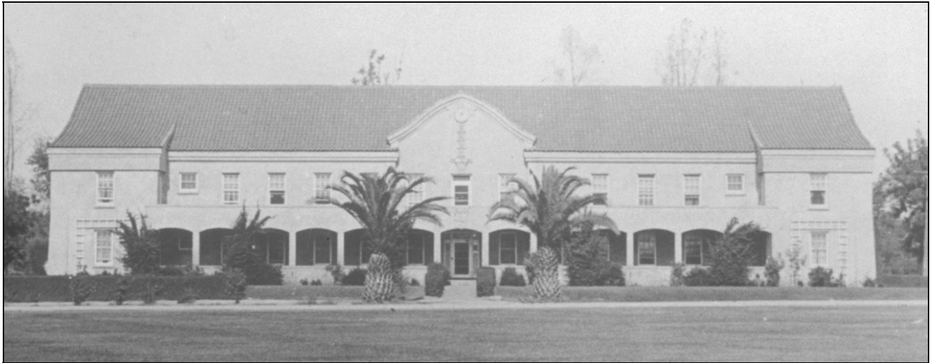
Figure 9: Undated photograph of Nurse's Home. Note presence of cast concrete ornament in gambrel dormer, multi-light windows, ornamental trellises around windows on east and west ends, and symmetrically planted palm trees. Photograph courtesy of UCD Medical Center Facilities Management.
