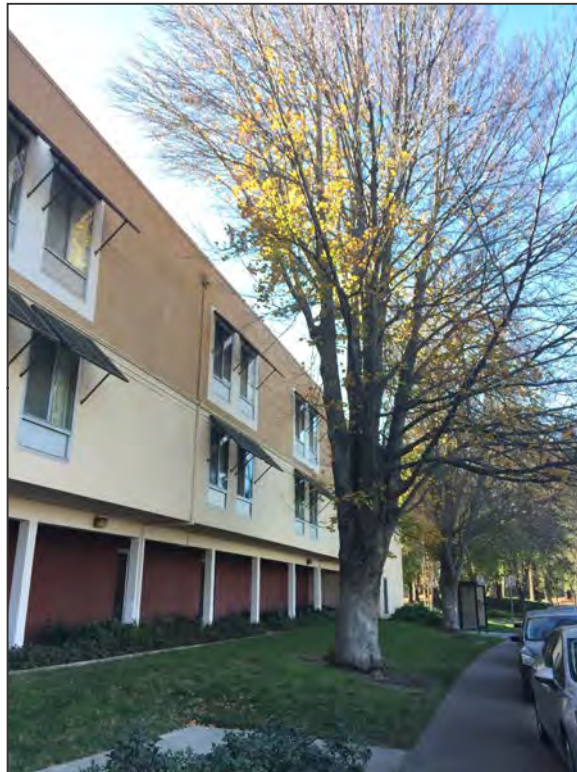
Looking west along the western side of Emerson Hall
