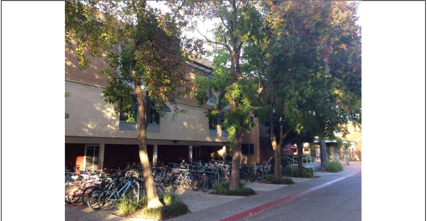
Figure 14. Main Elevation, View to Northeast, November 14, 2017 (IMG_0847)
