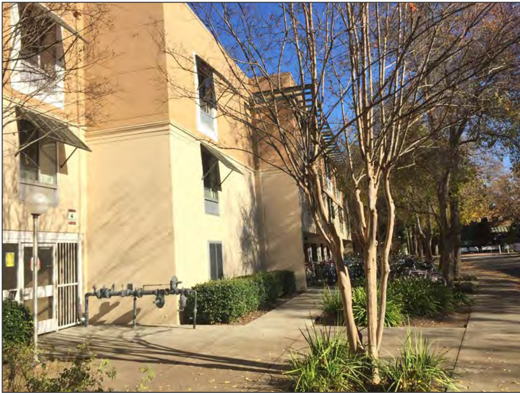
Looking east along the southern side of Emerson Hall
