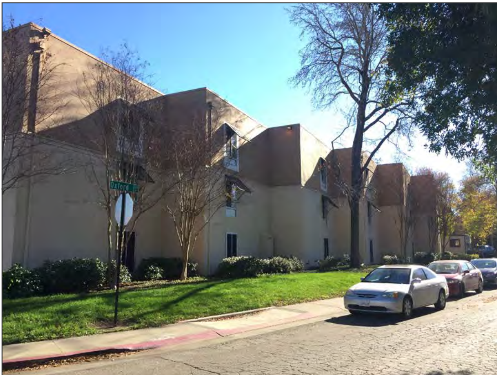
Looking south along the western side of Emerson Hall
